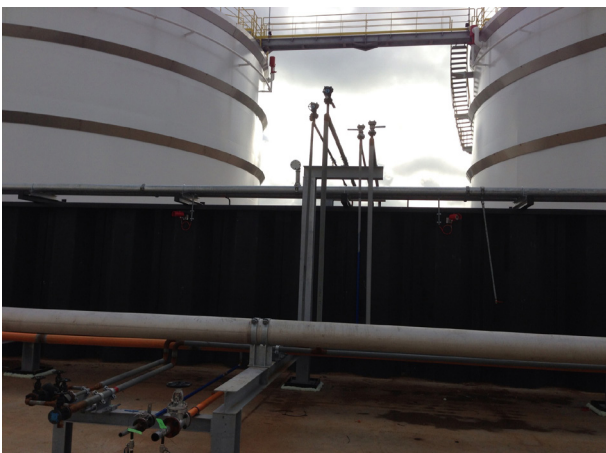
Figure 5. Flame detectors, such as Emerson's Rosemount 975 family, look for radiation in specific wavelengths emitted by hydrocarbon or hydrogen-based combustion.
