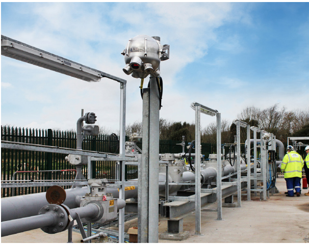
Figure 4. An ultrasonic gas leak detector, such as Emerson's Incus Ultrasonic Gas Leak Detector, can capture the sound of a compressed gas leak.
