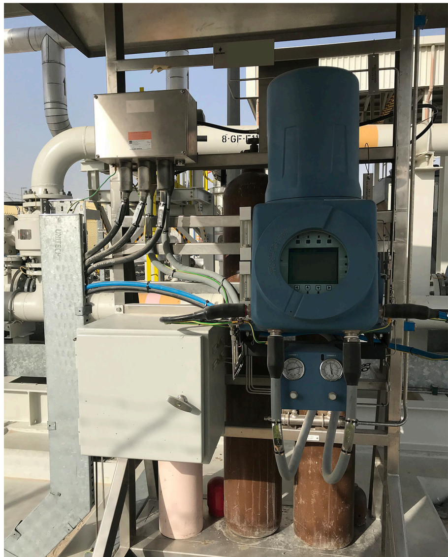
Figure 6. Detailed natural gas analysis calls for a C9+ analyser, such as Emerson's Rosemount 700XA Process Gas Chromatograph.
