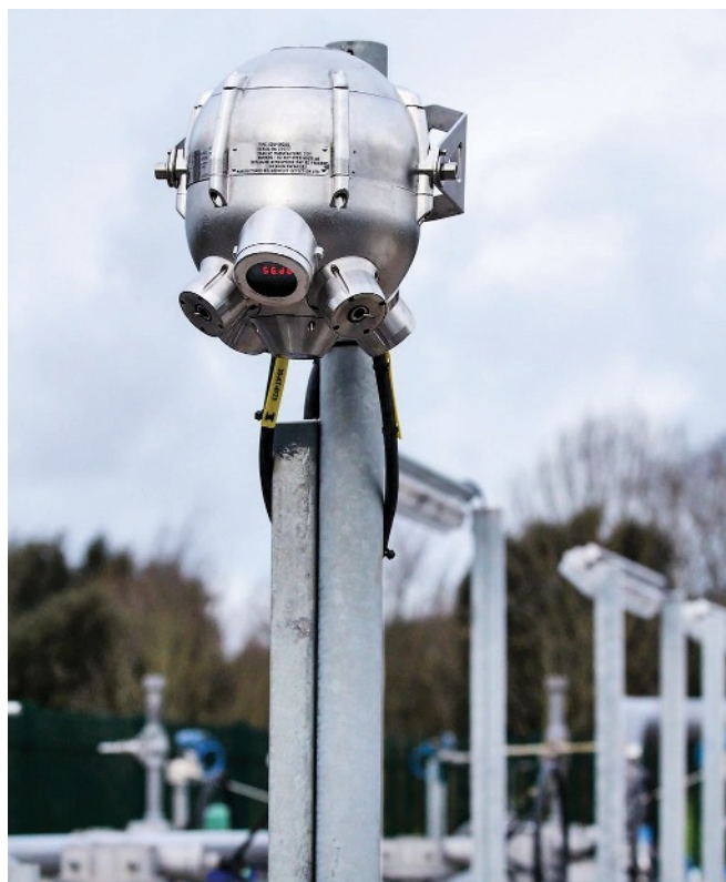
FIG. 3. Ultrasonic gas detectors do not look for a specific gas, but instead listen for characteristic noises made in ultrasonic frequency ranges by pressurized gas escaping through a leak. When positioned carefully, they can detect a release long before enough gas has escaped to be detectable by other methods. Photo courtesy of Emerson.
