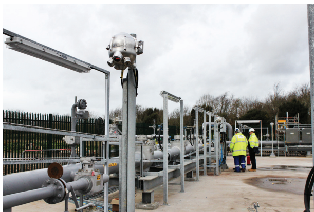
Figure 1. Ultrasonic gas leak detector.
