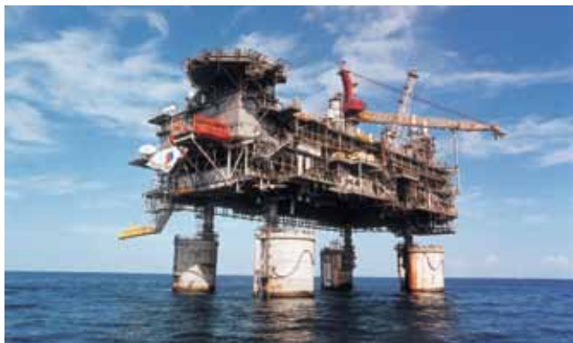
Figure 2: Instruments on offshore platform can be accessed from onshore facility.
