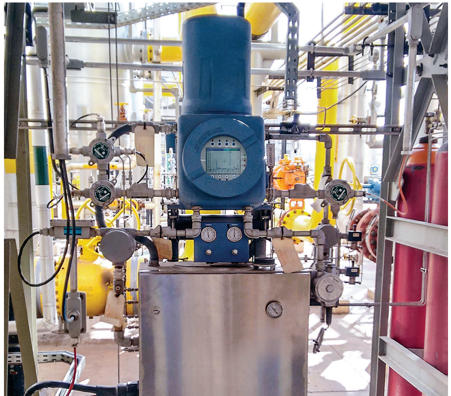
FIG. 1. Gas chromatographs are used to make a wide variety of measurements in ethylene plants.
