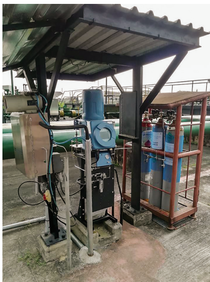
FIG. 5. Detailed natural gas analysis requires a C_9+ analyzer. 9
