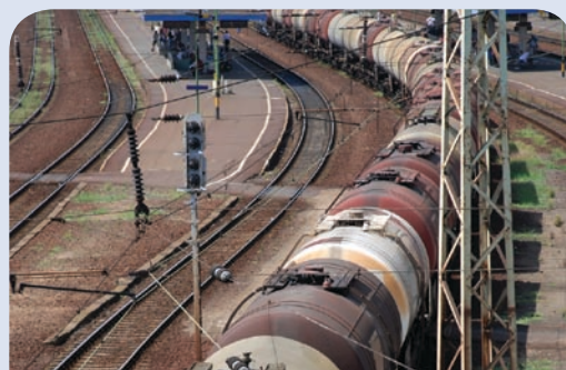
At Croda, wireless temperature transmitters help boost operator safety and efficiency.
