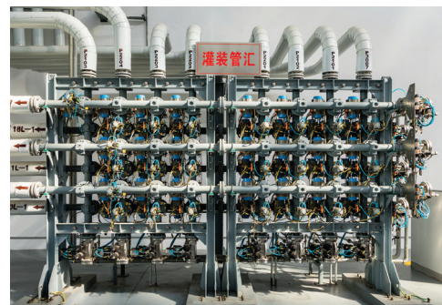
A finished product manifold equipped with 8 inlets and 6 outlets. Photo courtesy of Copton.
