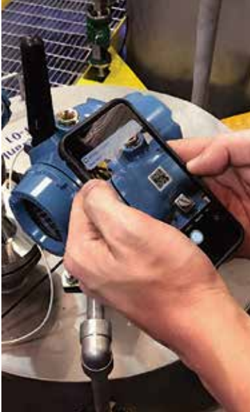
Scan the QR code on the device for serialized device information in the field.
