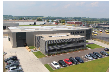
FIGURE 9 Emerson's AEV facility in Belgium
