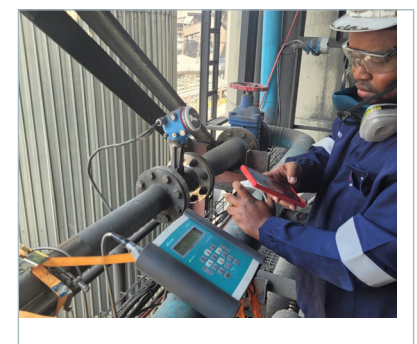
Control measurements with the portable FLUXUS® G601 on a compressed air line
