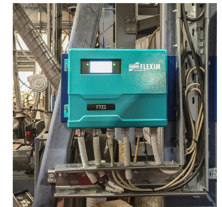
The stationary FLUXUS® F722 is used as the transmitter.
