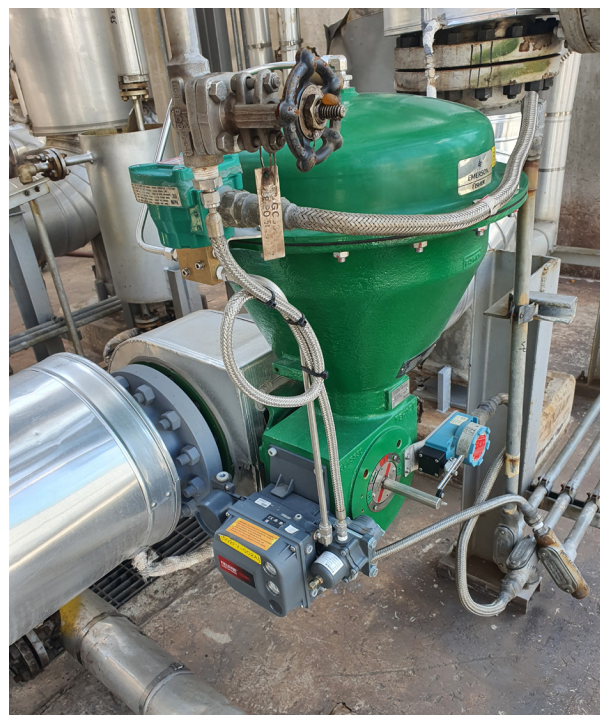
Fisher Vee-Ball Cavitrol™ Hex Trim combines the advantages of Vee-Ball capacity and rangeability with Cavitrol Hex Trim that helps prevent cavitation.
