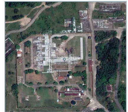
Aerial view of the Centro Comercializador de Crudo Palomas (C.C.C. Palomas), located near Coatzacoalcos in the State of Veracruz, Mexico. © Google Maps
