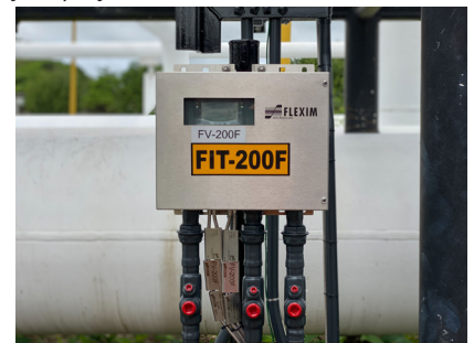
The stainless-steel version of the FLUXUS® H721 ultrasonic HPI measuring system is used as transmitter.
