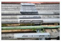
Measurement points next to the ships' stop. Installations without cutting pipes and without process interruption. This measurement point comprised 10 pipes with dimensions between 8" and 10". M and K transducers were used for this application.
