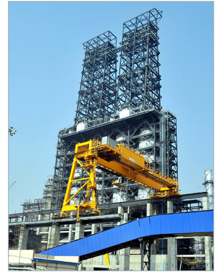
The Delayed Coker Unit (DCU) © HMEI
