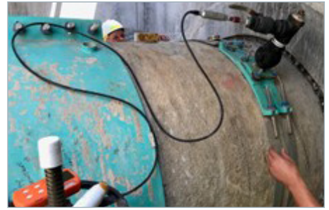
What insertion meters showed and what was actually measured coming out of the force main never aligned. Flexim meters more accurately reflect the expected flow.
