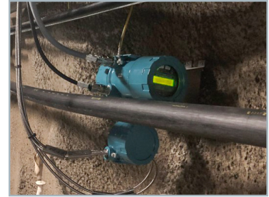
The FLUXUS® G809 was originally intended as the transmitter. Its channel switching proved to be too slow in some operating situations.
