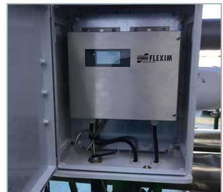
A stationary FLUXUS® F721 in stainless steel housing is used as measuring transmitter.
