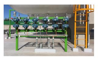
Data from each tank is sent over both the wired and wireless networks to the control room. This enables a very robust communication solution with built-in redundancy.
