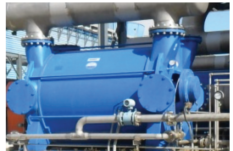
Installed Magnetic Flow Meter in a cooling water application.
