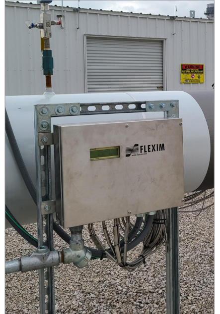
The stationary FLUXUS® G706 is used as a measuring transmitter.
