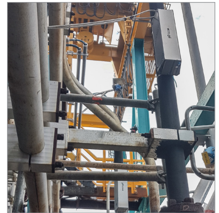
Two measuring points with the clamp-on ultrasonic transducers mounted in Variofix C
