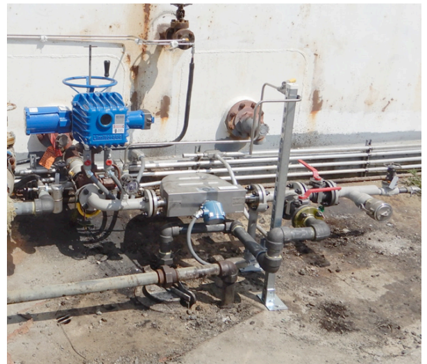
Fully automated configuration with valve actuator
