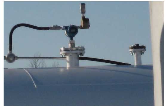
Figure 1. Installed Rosemount Smart Wireless THUM Adapter
