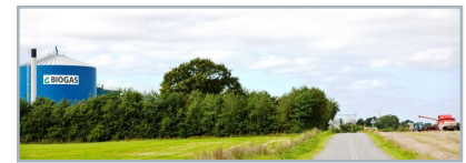
Bigadan's Sinding biogas plant
