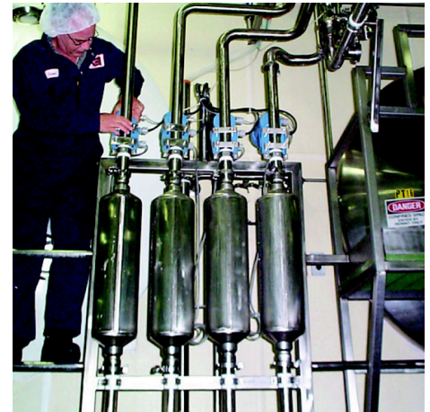
Installed Rosemount 8750WA Magnetic Flow Meter
