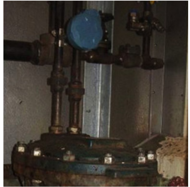
The Rosemount 708 Wireless Acoustic Transmitter features integrated sensors that mount externally to make installation fast, inexpensive, and non-intrusive to the process.
