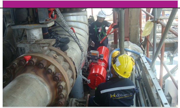
Emerson's channel partner Matco Thailand conducting a thorough site walkdown and overhauling six Bettis actuator units.
