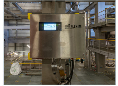
The stationary FLUXUS® G722 ST with stainless steel housing is used as the measuring transmitter.
