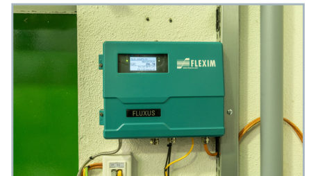
The stationary FLUXUS® G721 ST-LT with pressure and temperature compensation is used as the transmitter.
