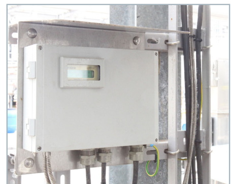
Stationary FLUXUS® F704AN ultrasonic measuring systems are used as transmitters.
