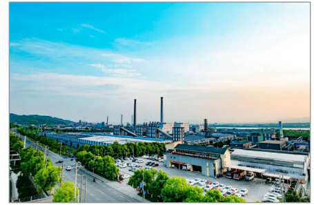
Overview of Hubei Yihua's chemical and fertilizer complex on the right bank of Yangtze river
