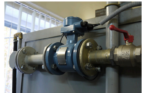
Rosemount Magnetic Flow Meters measure water and foam agent flow rate in fire engines with a capacity of up to 200 liters per second.
