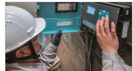
The final parameterisation of the FLUXUS® F721 stationary transmitter is a routine task for the experienced service engineer.
