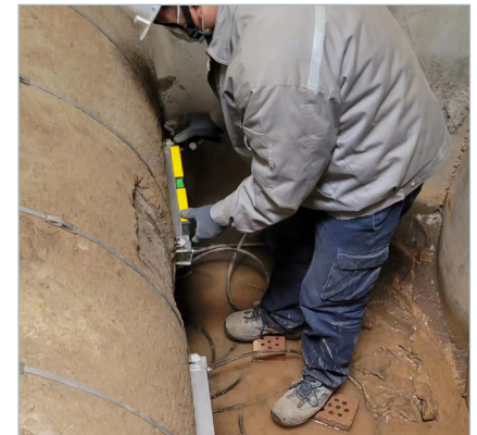
After the service engineer has determined the most suitable measurement location with his portable FLUXUS® F601, the clamp-on transducers are permanently installed there on the outside of the pipe with Variofix L mounting rails.
