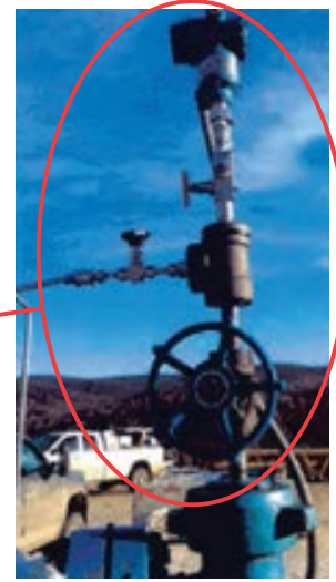
Vertical install - Qty 1 chemical injection line Fully assembled and tested in Harlingen, Texas - USA
