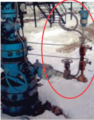
Horizontal install - Qty 2 chemical injection lines
