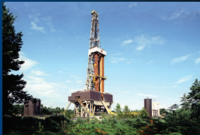
Wireless installation made easy. (Image courtesy of BP)
