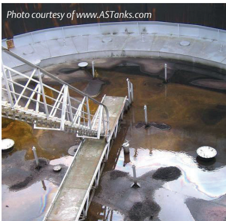
Improper draining can severely disturb roof operation.
