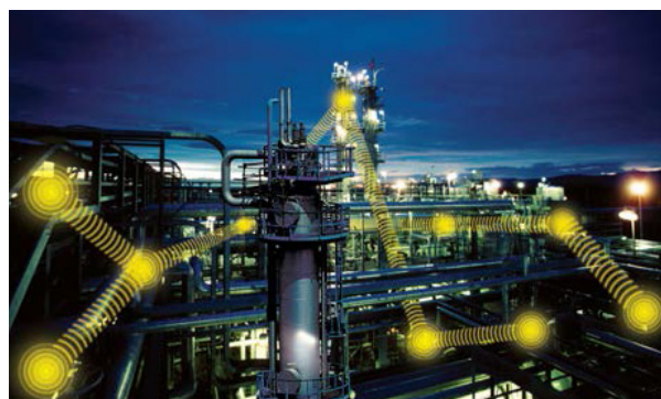
Emerson Smart Wireless Temperature Transmitters form a self-organizing wireless network across the Jubail plant.
