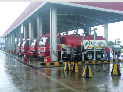
Terminal Truck Loading
