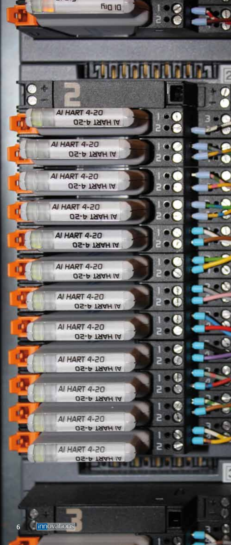
Left: The secret to Electronic Marshalling is a device called a CHARacterisation Module (CHARM).
