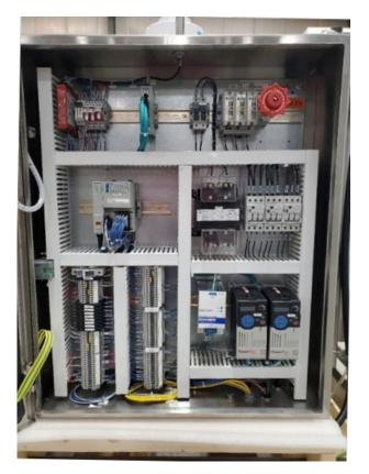
The panel contains the following key components: Safety control circuit, network hub, isolation switch, PLC, 3 phase to single phase transformer, Power supplies, and conveyor drives.
