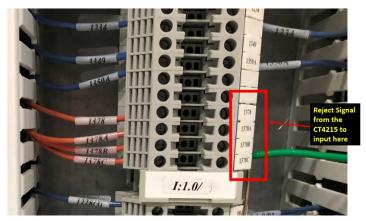
3. Disabled – The reject station can be disabled by not providing reject signal from the CT4215 base system.
