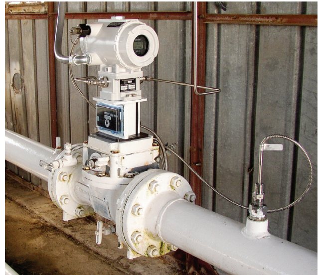
Figure 3. FloBoss™ 104 The FloBoss™ 104 is a cost effective flow computer for either rotary or turbine metering.
