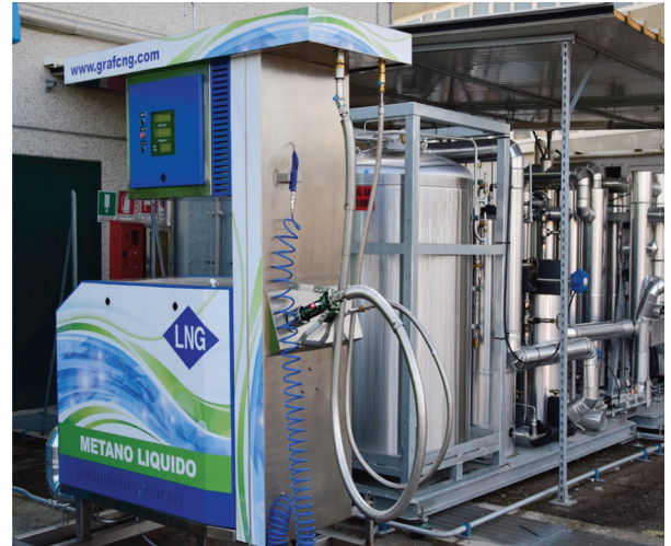
The complete solution from Graf includes liquification, storage and dispenser
