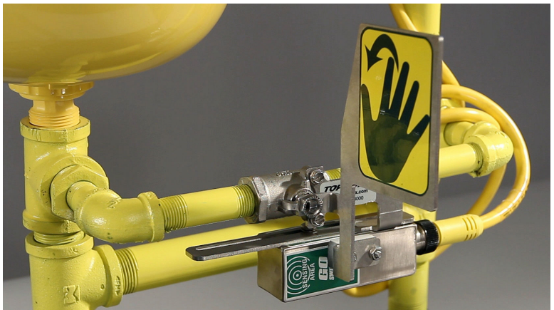
Figure 7-2: TopWorx Switch Installed on an Eye Wash Station
