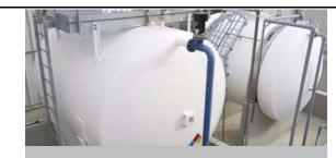
The low frequency of the Guided Wave Radar products ensures reliable level measurements in vessels with vapors such as anhydrous ammonia.
