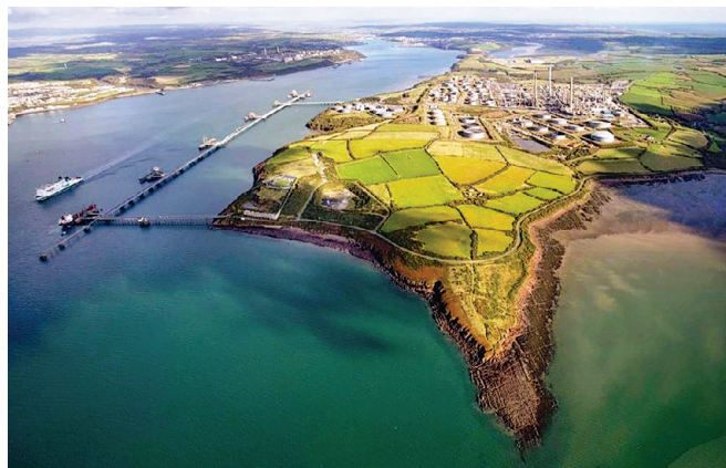
FIG. 1. The Pembroke refinery in Wales has eight berths for ships and more than 100 tanks of various sizes with total capacity of 10.5 MMbbl.
